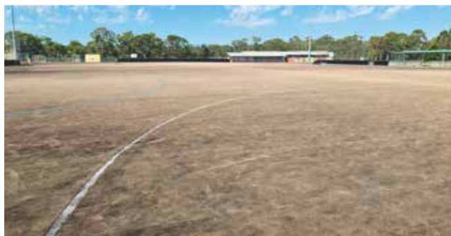
Above: Cessnock Baddeley Park Hockey Field current surface was severely damaged due to flooding events.
